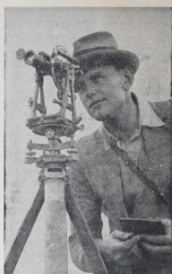
THE SURVEYOR.—A surveyor engaged in Napier geodesy.
