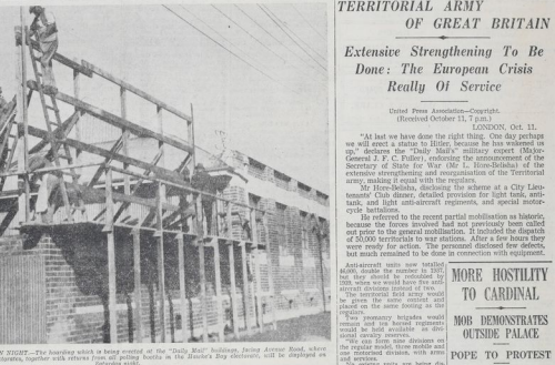
PREPARING FOR BARRAGE BOMBING. The building which is being erected by the 'Daily Mail' building, being erected here, when it is completed will be the largest building in the city.
