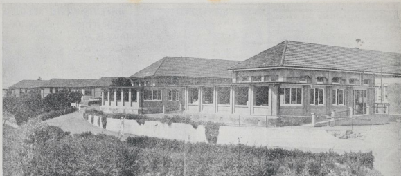
A photograph taken by the "Daily Mail" cameraman yesterday of a section of the Napier Hospital. Situated high on the hills overlooking Napier and its suburbs, attractive grounds, the hospital is a well known landmark.
