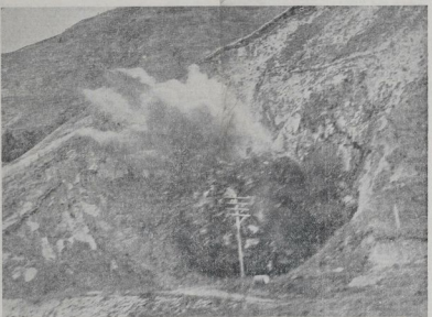
TWO THOUSAND POUNDS OF GENUINE BRICK BORN FROM YARDS OF ROCK AT KAPER'S QUARRY, NEAR PORANGAKA, FEBRUARY 20, AFTERMATHS OF THE "Daily Mail" explosion in Hastings after the charge had been fired. Some one of the men of the party of rock men through the dust can be seen by comparison with the rubble in the foreground. The contractor was Mr. Henry Anderson, of Napier, and he said he was not in the quarry at the time of the explosion.
