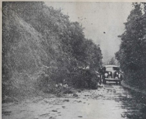
ONE OF THE MANY SMALL SLIPS WHICH CAME DOWN IN THE MANAWATU GORGE DURING THE STORM.
