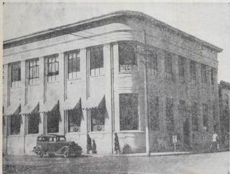
DALGETY'S BUILDINGS, DICKSON STREET, NAPIER, where the studios are situated.
