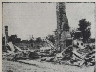
PARADES FIDE. —The ruins of a Turakou house which was destroyed by fire on Monday night.
