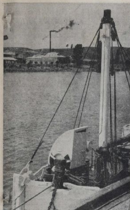
ACROSS THE RIVER. —A pier goes at Waimea, with the piling works in the background.
