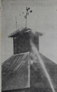
HASTINGS BREWERY FIRE —Hot iron buckles under the force of water from the hose, while the water-tower remains protected from fire.
