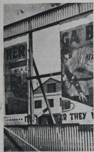
CRASH!—An entire road in a large housing near the Hastings Exchange Station was blown out during the heaviest of yesterday's gales.
