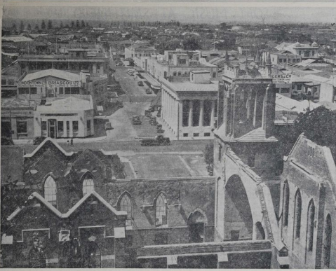
AN UNUSUAL VIEW OF NAPIER.—Looking across the ruins of the Presbyterian Church, which was destroyed in the 1931 earthquake by the evergreen suburbs to the north.
