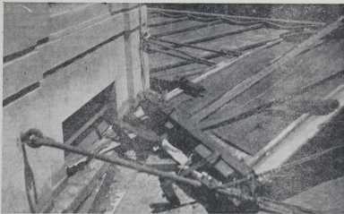
TIIPPED OFF BY THE WIND.—The remains of a heavy iron sign, 3ft. dia. by 6ft. dia., which was ripped off a theatre wall to which it was attached by heavy bolts, by the force of the wind on Napier on Monday morning.
