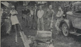
AT LAKE TUTIRA.—New telephone boxes are being erected in the Tutira district. This photograph shows a bathroom's view of the edge of the lake.
