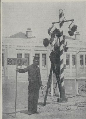
THE STOP AND THE LIGHT.—One of the new traffic signals which have been installed at the St. Andrew Street military crossing, Hastings. The signals will replace the old portable "stop" signs.
