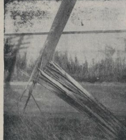
POLE INTO WATERHOOD.—This telephone pole near Lennox Park, Hastings, appearing when it was struck by a motor-car on Saturday morning. None of the four occupants in the car escaped injury, while the fourth suffered a cut.
