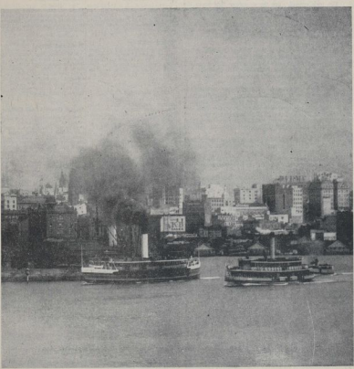
CANADIAN QUEEN.—A view of Canadian Queen with port of her motor installed since in the background. A contract is now under way for the reconstruction of the Canadian Queen waterfront.
