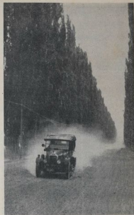
ROAD RECONSTRUCTION —Motorists who have suffered from the clouds of fine dust in Poplar Avenue, Ashburton, will be glad to know that the dust situation will now be cured.
