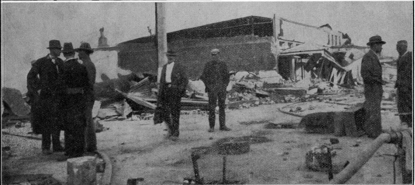
Hastings—Above—Wrecked premises in the main street. Centre—All that was left of Roach's store. There were fifty people on the top floor at the time of the earthquake, and it is known that nine of the girls employed lost their lives. Below—Odd cases of looting occurred, and the picture shows the patrols guarding the ruins against further thefts.
