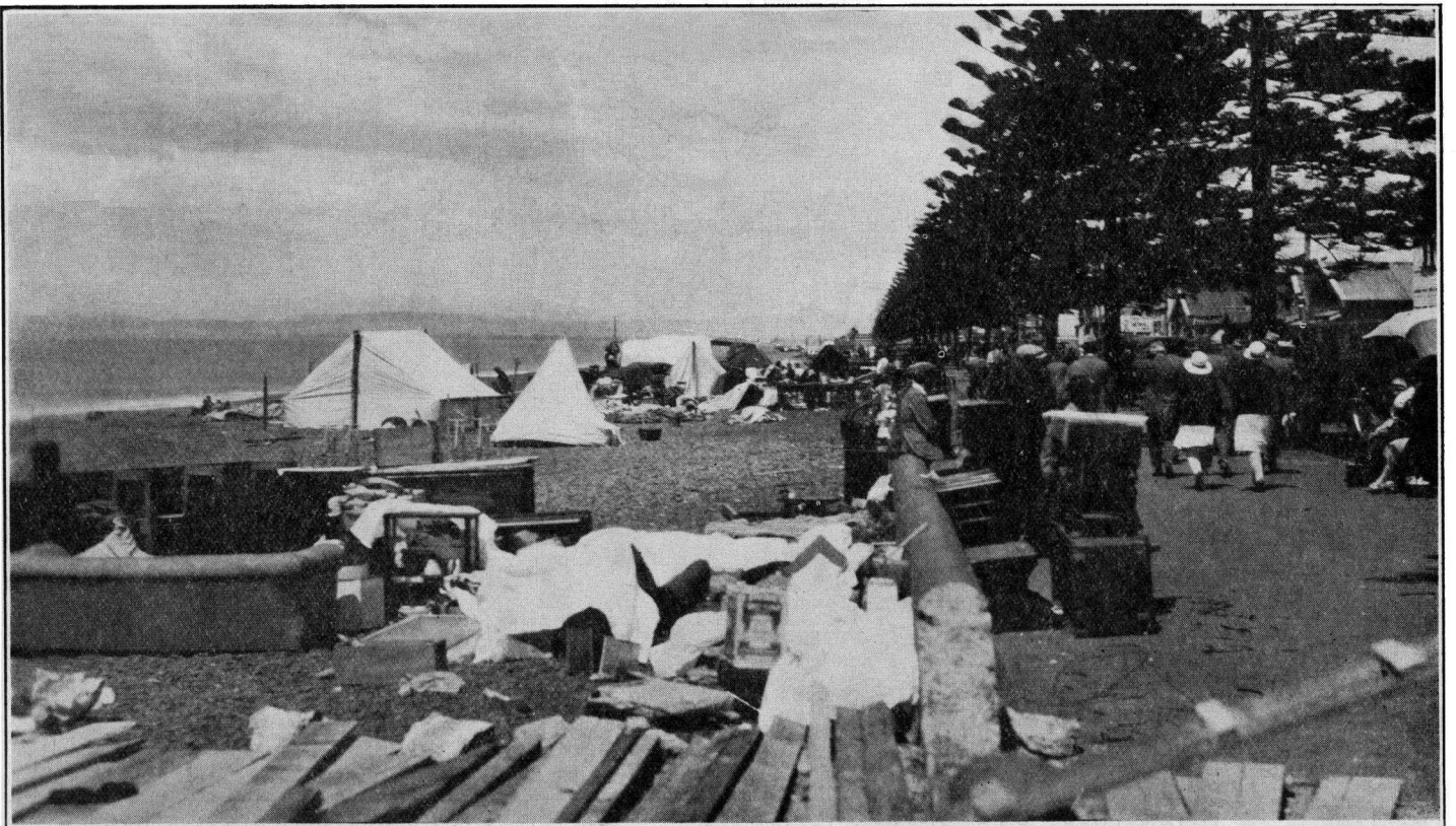
Napier—With their homes gone and with gaunt fear in their hearts, making them afraid to sleep inside buildings, thousands of people spent the nights on the sea shore in tents and under all manner of improvised structures.
