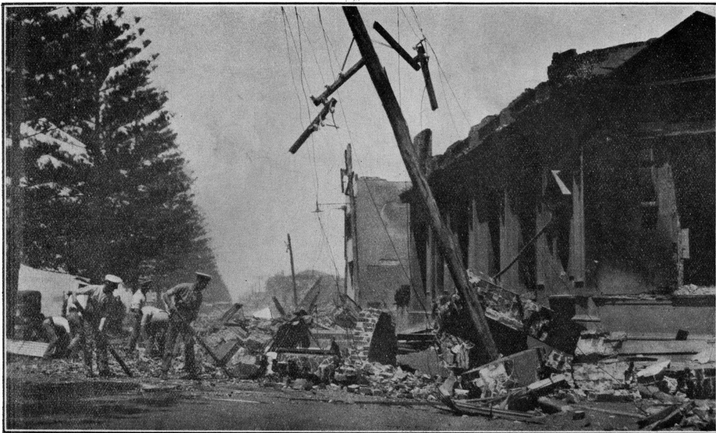
Napier—Looking along the Marine Parade, once the pride of the town. The photograph shows the remains of Messrs. Murray, Roberts and Co., Ltd.'s building and that of the Y.M.C.A. Bluejackets from the warships can be seen searching among the remains for bodies.
