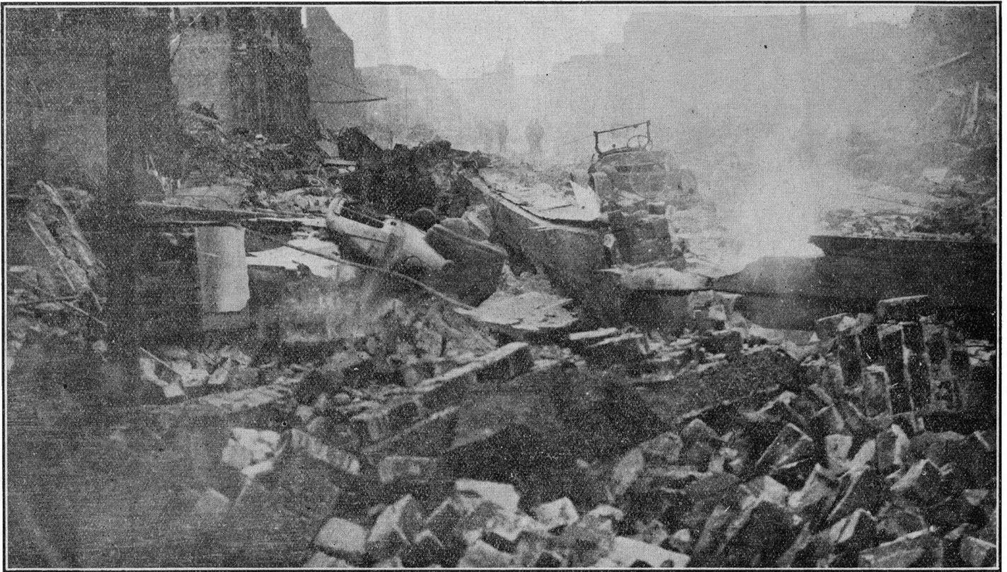
Napier—An illustration giving an excellent idea of the utter wrecking of the buildings, and showing how little hope there was for those unfortunate people caught beneath the falling walls.
