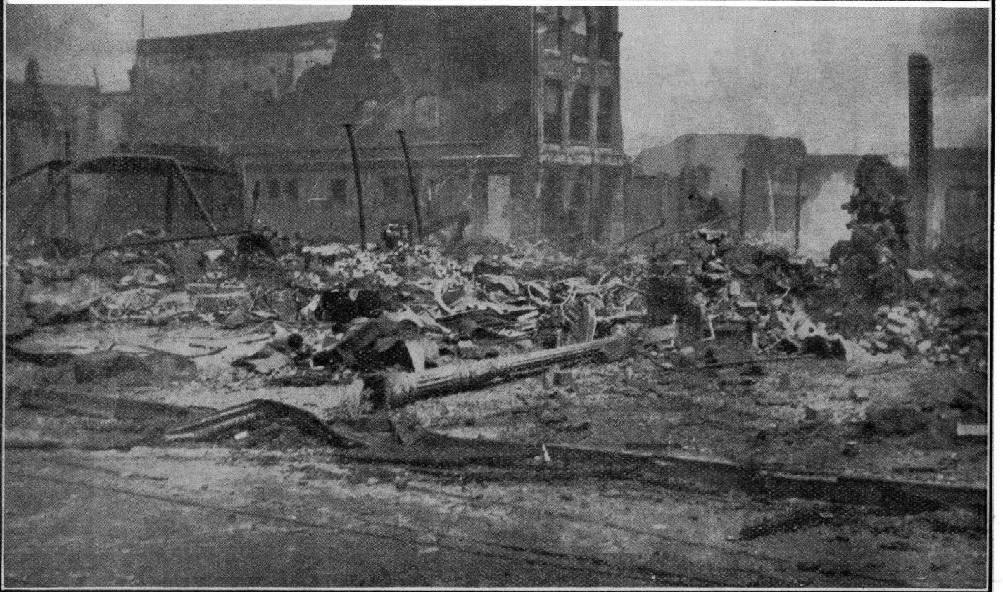
Napier—Giant masses of masonry were taken and thrown about as though they were pebbles. Note the two blocks in the picture above. Below is another picture taken while the fires were ravaging what the earthquake left behind in its track.
