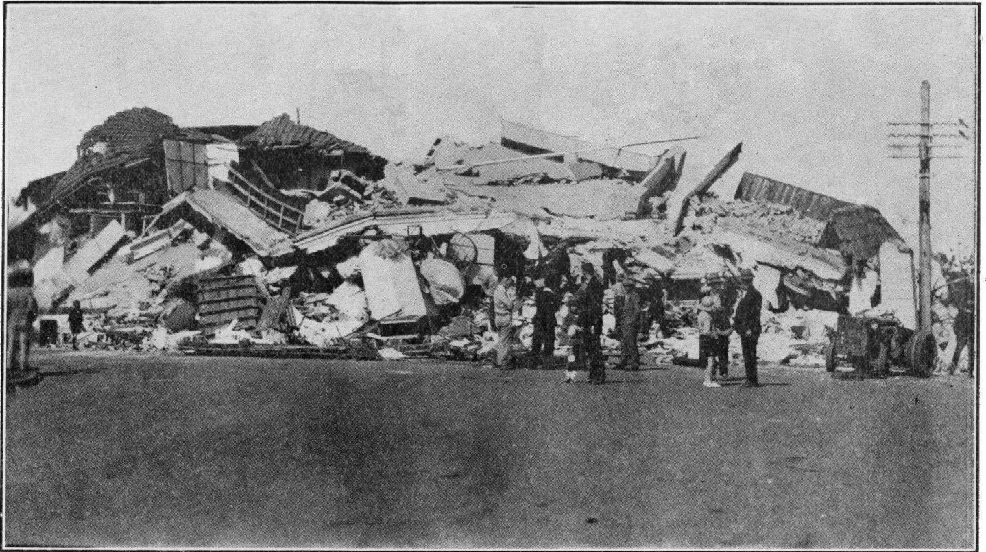
Napier—One of the greatest tragedies happened in this building—the Nurses' Home at the Hospital. Here Sisters and nurses were crushed while they were lying in bed. Reference to the heroic action of those saved is made in the text at the beginning of the issue.
