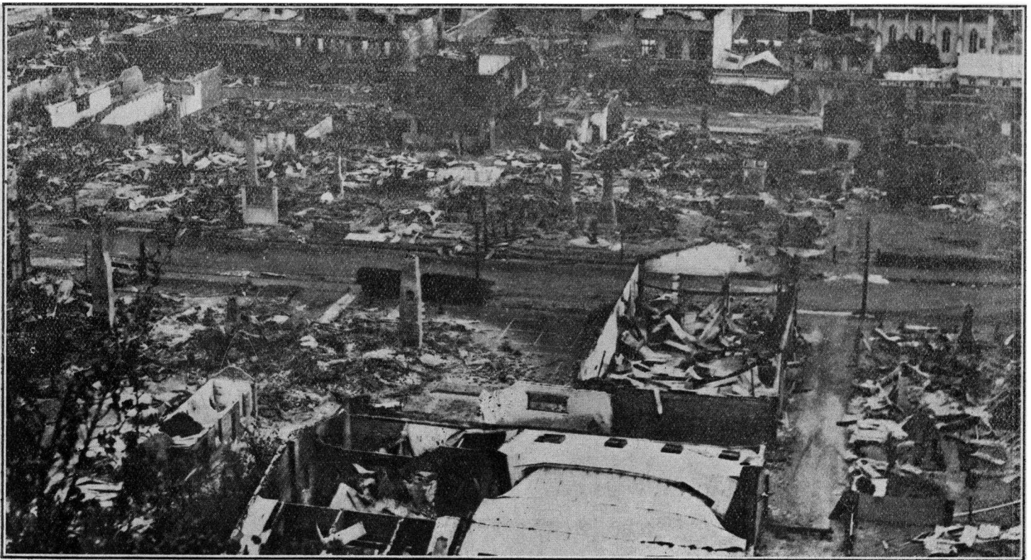
Napier—After the fires had died out. The main business area, where it is estimated that the damage will reach in the vicinity of £9,000,000.
