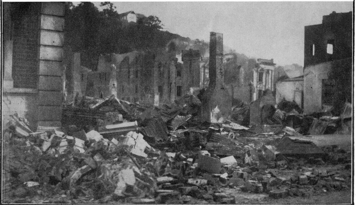
Napier—Street after street is the same. These remarkable photographs show in detail the damage done in the stricken area. One of the curiosities is the fact that some chimneys remained standing through it all.
