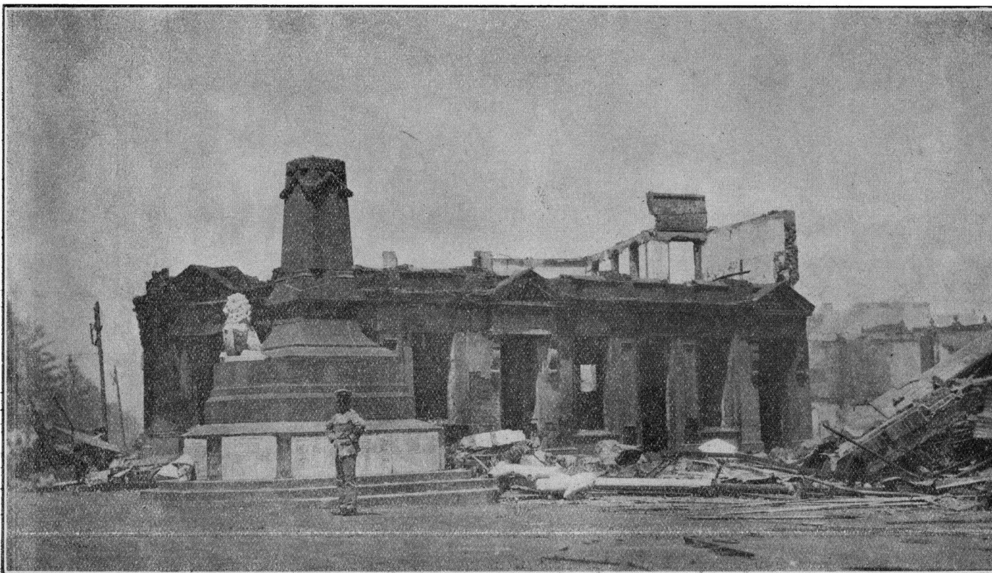
Napier—In the foreground can be seen all that remains of the fine memorial erected to those who fell in the Boer War. At the back is all that is left of a fine building.
