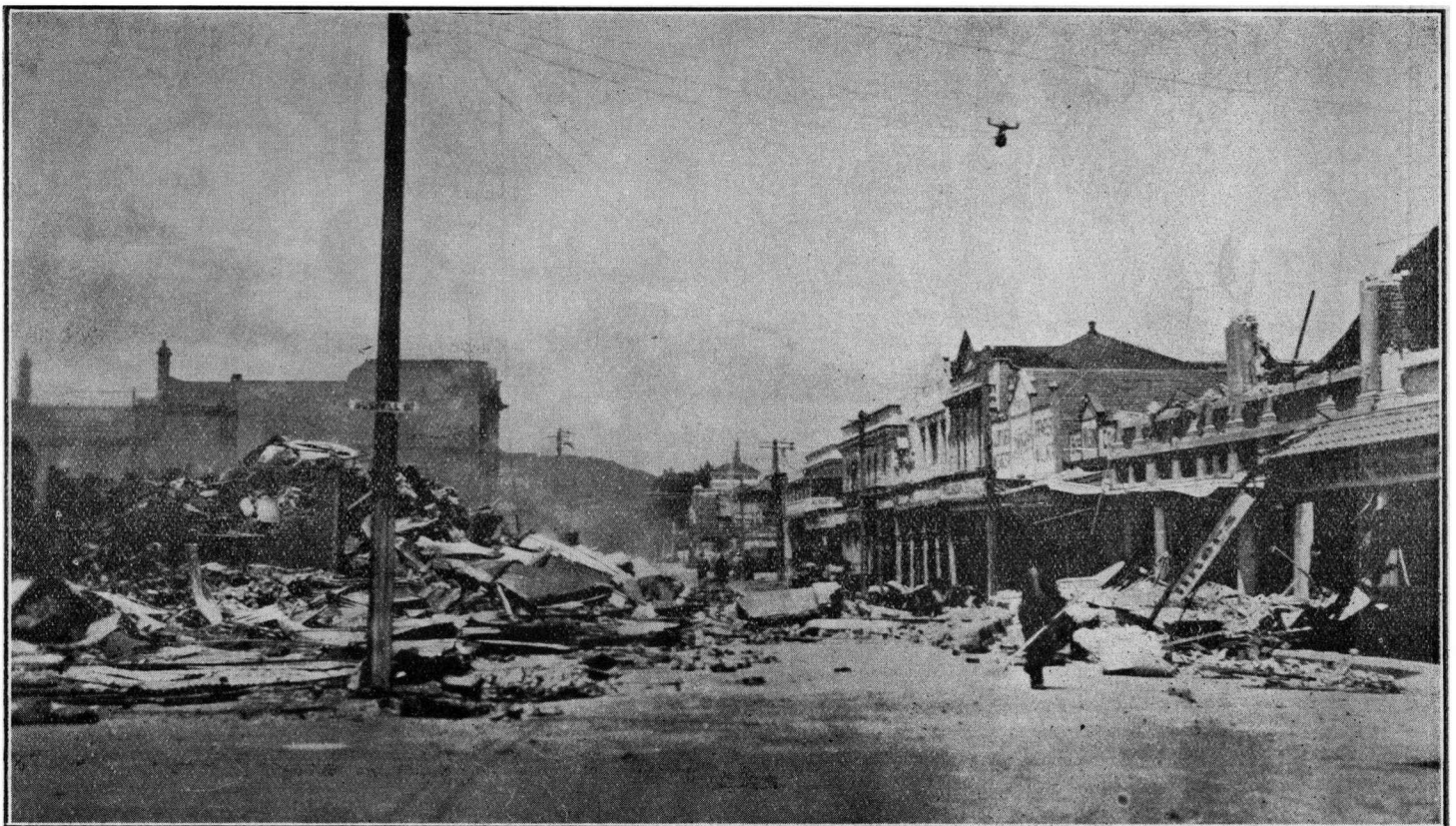
Hastings—Looking from Russell Street along the length of Heretaunga Street. The buildings on the left-hand side of the photograph have been completely wiped out.
