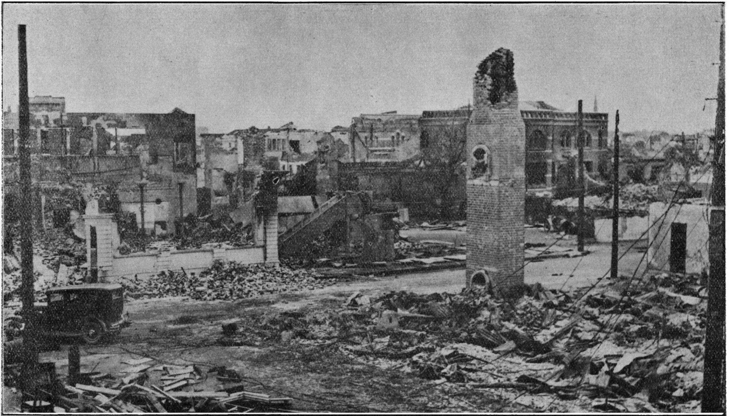
Napier—A mass of tangled wires and debris strewn about the streets. Another scene in the business area.
