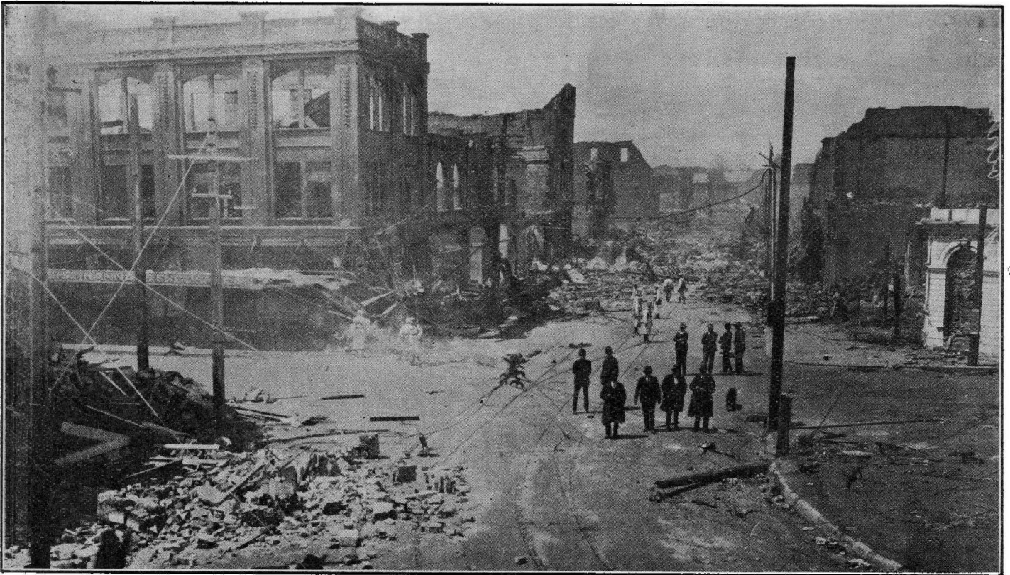
Napier—Looking down Hastings Street, where the wreckage completely blocked the thoroughfare. On the right is all that is left of the Bank of New Zealand building.
