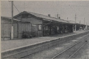
WANTED.—A new station for Hastings. Representatives to the Government are continuing to have the building replaced by a modern structure in keeping with the needs and progress of the district.
