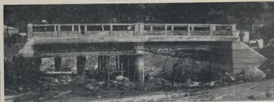
HARVESTING WATER AT WAIKAREMOANA. —The new spillway weir at Waikaremoana, which is nearing completion, will enable an abundance of water to be used for power purposes.
