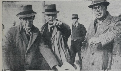
PLANS AND DISCUSSIONS —The general manager of New Zealand railways (Mr G. H. Mackley) discusses details of the East Coast rail service and the official opening on Saturday next. At right is Mr A. Dwyer, Public Works engineer-in-charge, Napier.
