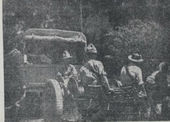
REGULARS WITH LOCALLY MECHANISED CABLE LAYERS.
