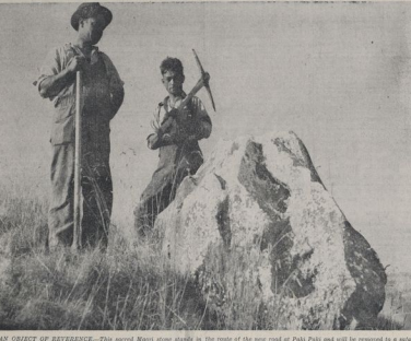
AN OBJECT OF REFERENCE.—The second stone above stands in the center of the new road of Park Place and will be removed to a new site.
