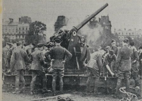
LONDON'S AIR DEFENCES.—Fortified have been busy for several months in the organization of anti-aircraft defences in and around London. Work of this nature has been greatly expedited up during the last few weeks.
