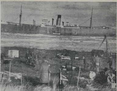
A CRITICAL AND ANXIOUS PERIOD. —The back of Charlton's home with extensive sea preparations are made for salvage operations where the Port Bowen is stranded. The construction between ship and shore are maintained by the lighters and the three jacks above. Water is supplied to the ship by the line.
