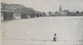
BRIDGE OVER THE TATARSKA—Warsaw has three bridges which span the Vistula, on which the city is situated. This is the largest of them. It is supported on five massive piers.
