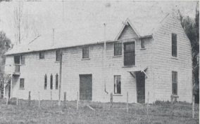
ONE OF THE OLDEST BUILDINGS IN HAWKES BAY —Formerly a hospital, this structure has been converted into a women's hall—St. Barnabas, Portland, Queen's Hill of the Anglican Church.
