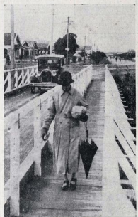
KENNEDY ROAD BRIDGE.—A view of the Kennedy Road across over the old Napier River. It is proposed that this bridge should be replaced by a modern one, with a new bridge to be replaced. It is proposed that this bridge should be replaced by a modern one, with a new bridge to be replaced. It is proposed that this bridge should be replaced by a modern one, with a new bridge to be replaced.
