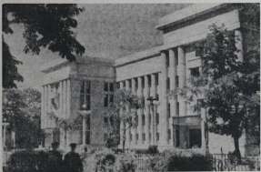
RED ARMY HEADQUARTERS —The Red Army directed its attack on Poland from this imposing building in a powerful offensive. Disrupters are located in block, a town with a population of about 350,000.
