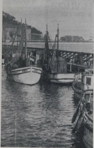
DISMISSED PROP—An October 25th, Captain James Cook first set foot on New Zealand and in Poverty Bay. The spot is marked by a monument, which is just visible in the background of this picture. Below, there is the ornate propeller of the ship which was the property of the Māori people. The heavy works on the left, and the screw propeller, which has been discarded, is at the right.
