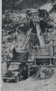
ROAD PROCEEDINGS FROM HILDESHEIM. —The regulations of the new approaches to the Tararua Bridge include removal of spoil removed from the face of the old works. Gravity chutes assist in loading operations.
