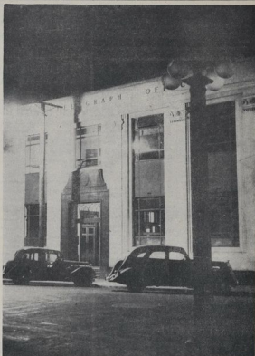
NO FLOOD-LIGHTS REQUIRED.—One of the new sunnery repair lamps hangs across the avenue before the Hastings Post Office facade.
