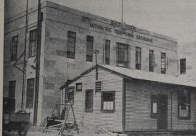
THE OLD AND THE NEW —The familiar temporary wooden board premises in Hester will now give place to the massive new structure behind, which houses the automatic systems for telephonic communication.
