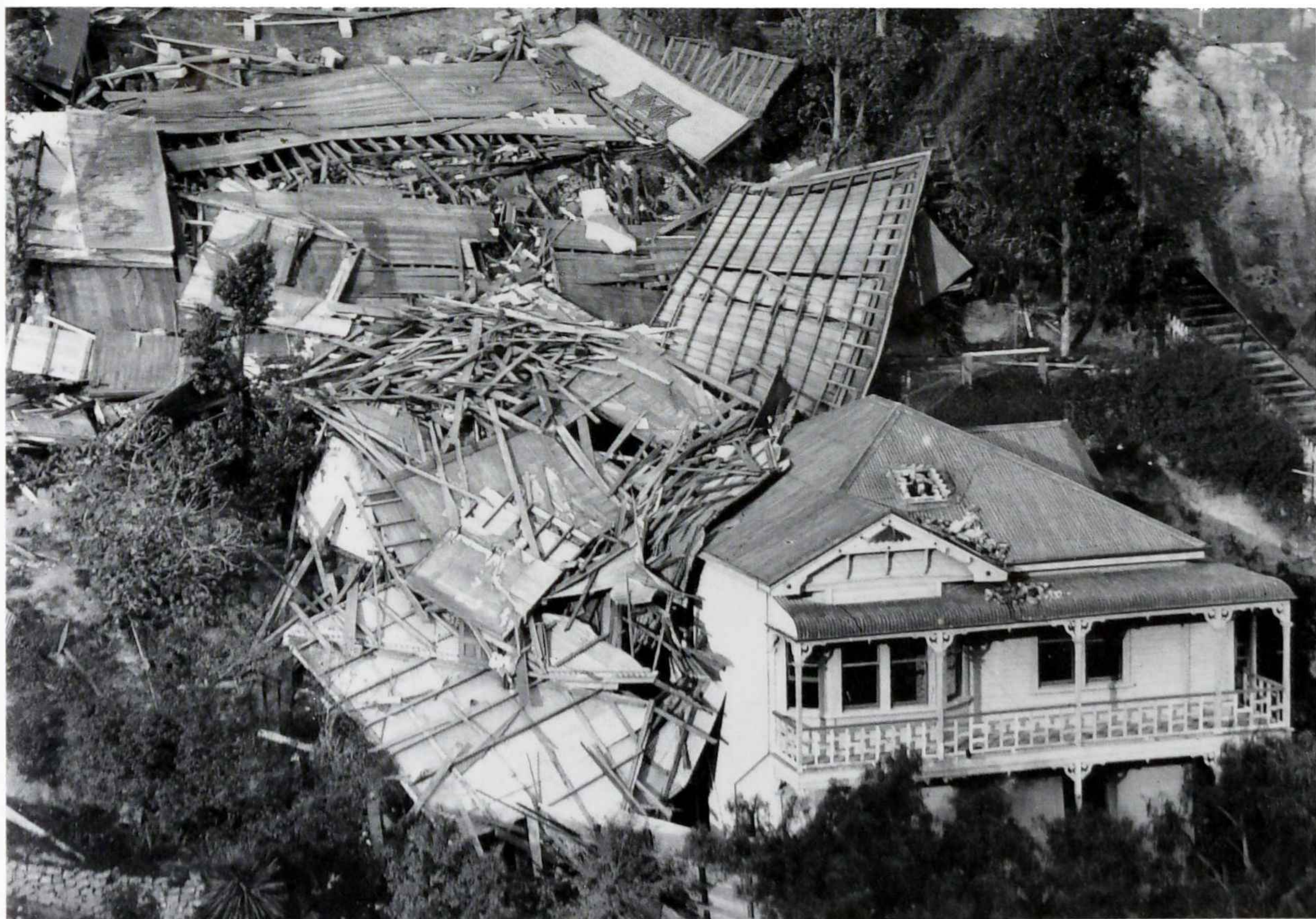
Wooden houses were rarely damaged severely, but this was an exception, jumping off its piles and cascading down the hillside. Its site, above Faraday Street, is still vacant.
