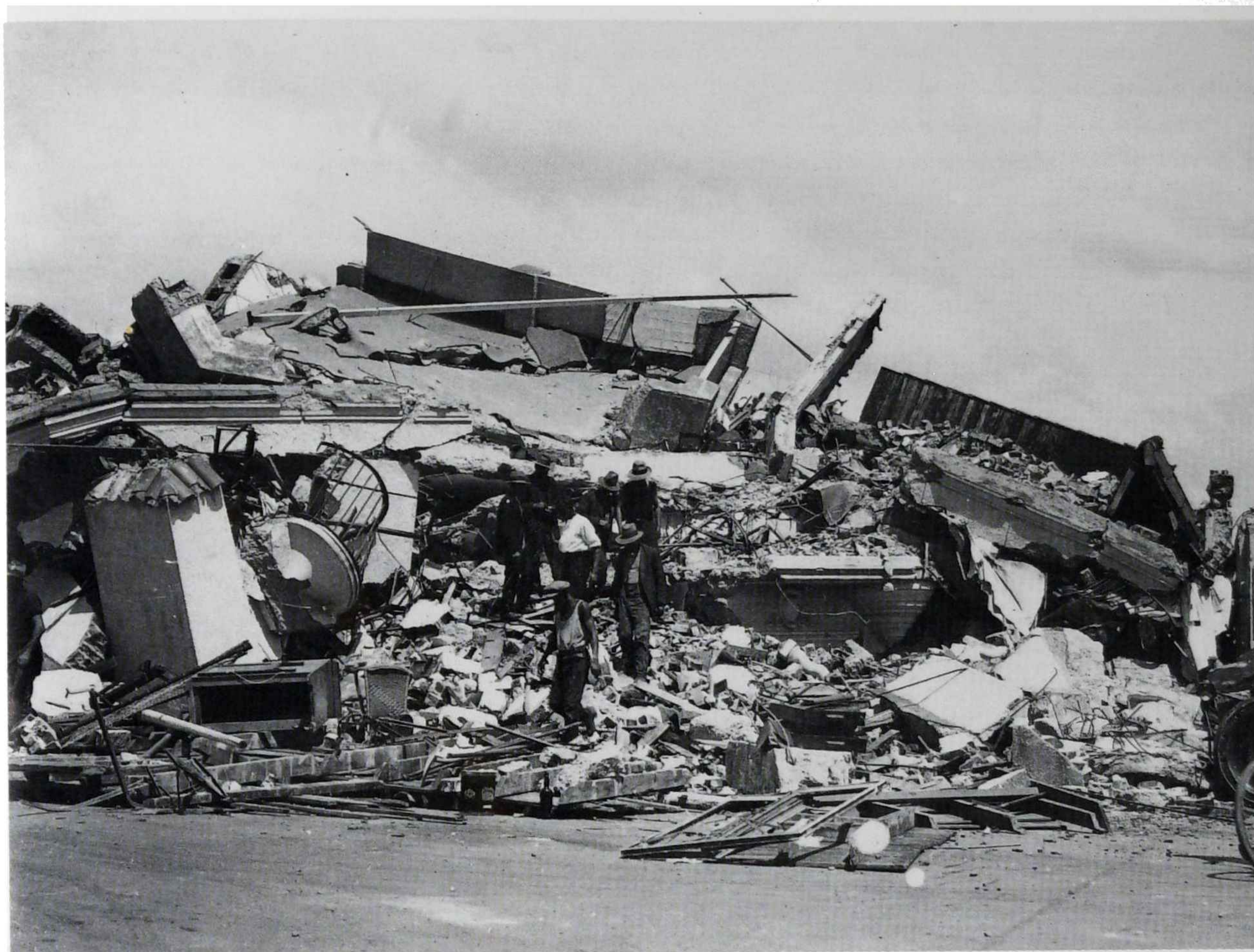
The appalling remains of Nurses' Home, in which several nurses died, asleep after being on night duty. An enquiry into its collapse found it faulty in both design and construction.
