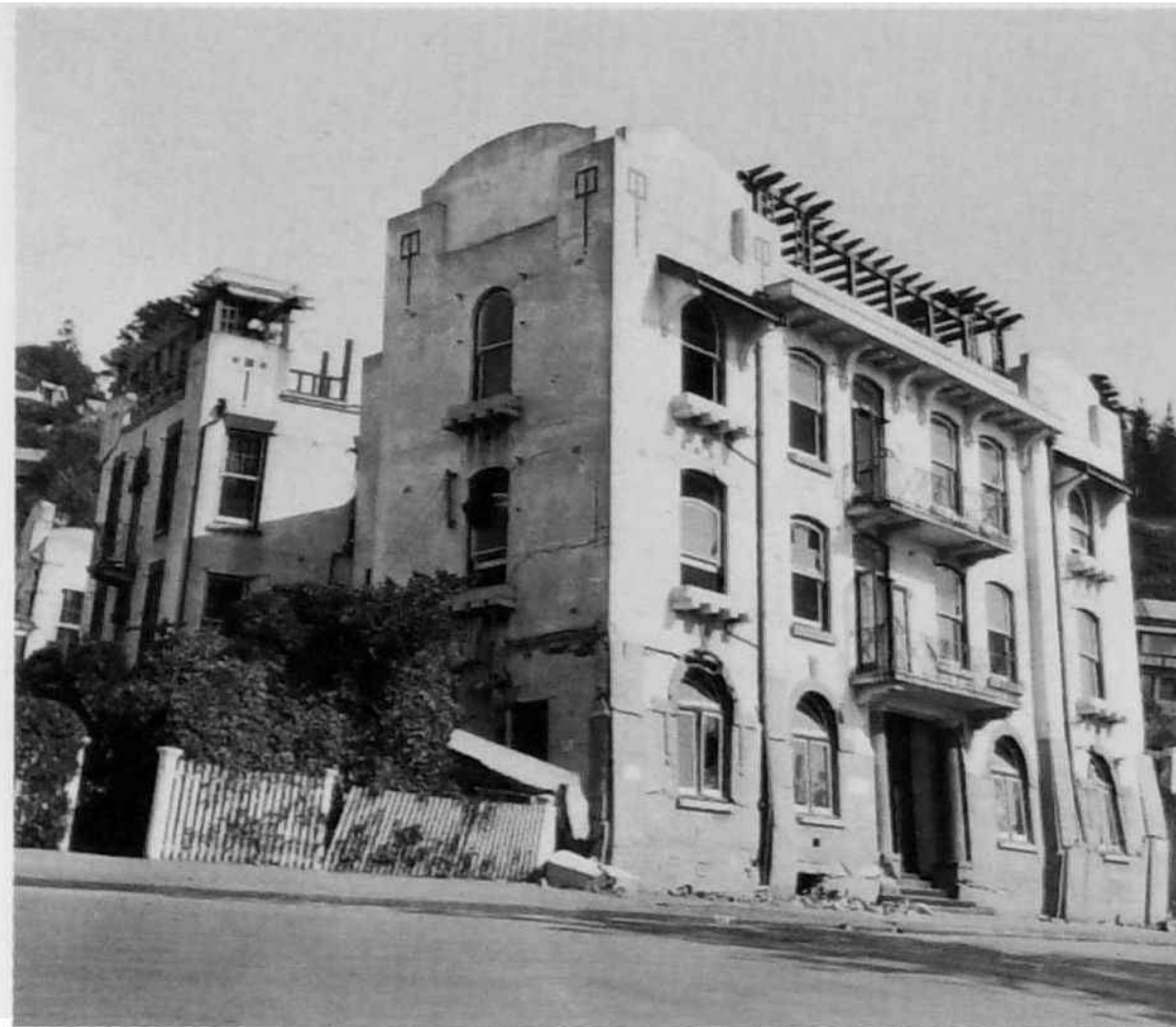
Dr Moore's Hospital tilted badly, crushing its mid-section. The damage was the result of excavations for an underground car-park, undertaken without engineering advice.
