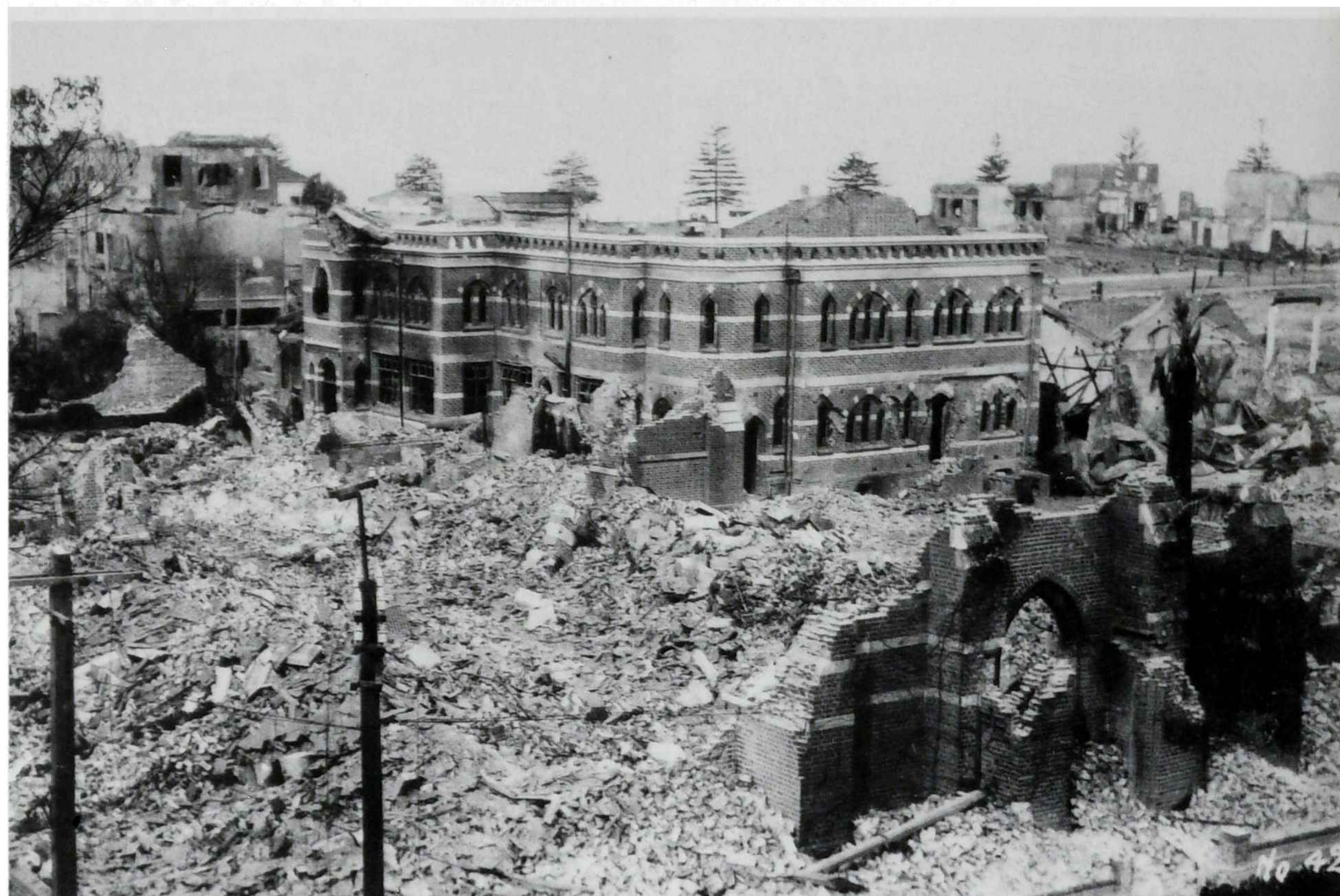
A pile of bricks was all that was left of St John's Cathedral. The Diocesan Offices behind, also built of brick but with reinforced concrete tie beams, were gutted by the fire but were still structurally sound.
