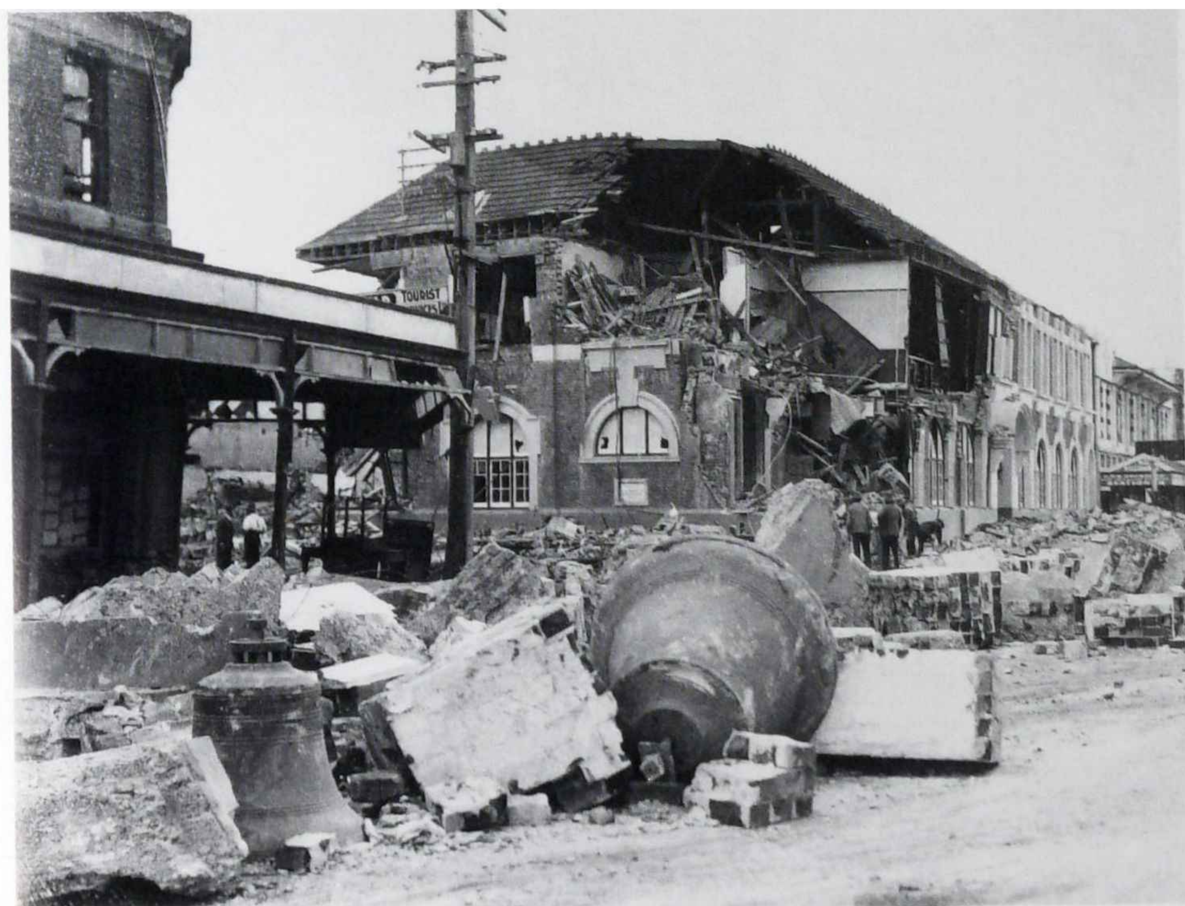
The appalling remains of Nurses' Home, in which several nurses died, asleep after being on night duty. An enquiry into its collapse found it faulty in both design and construction.
