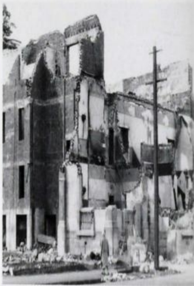
A pile of bricks was all that was left of St John's Cathedral. The Divesan Offices behind, also built of brick but with reinforced concrete tie beams, were gutted by the fire but were still structurally sound.
