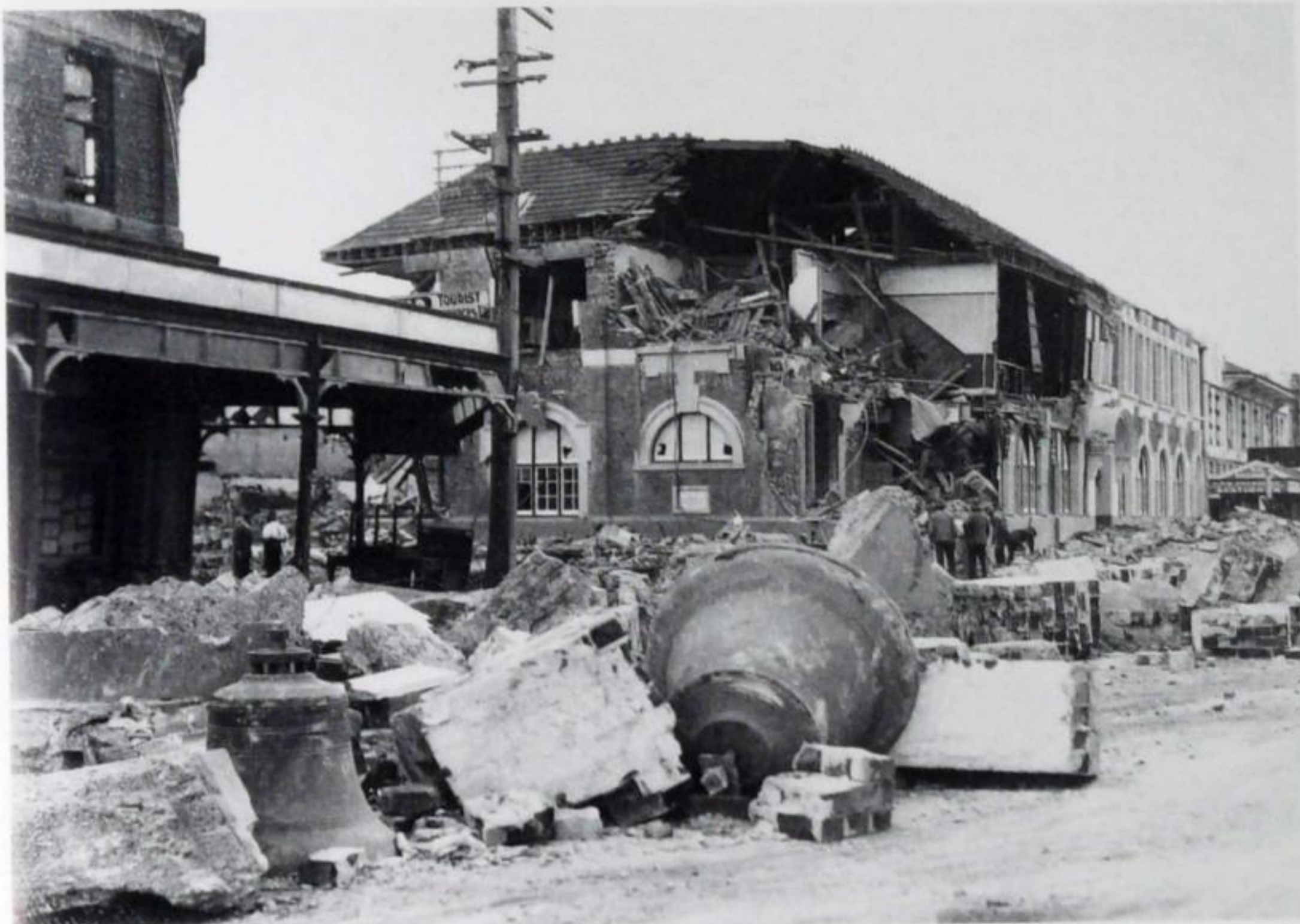
The appalling remains of Nurses' Home, in which several nurses died, asleep after being on night duty. An enquiry into its collapse found it faulty in both design and construction.
