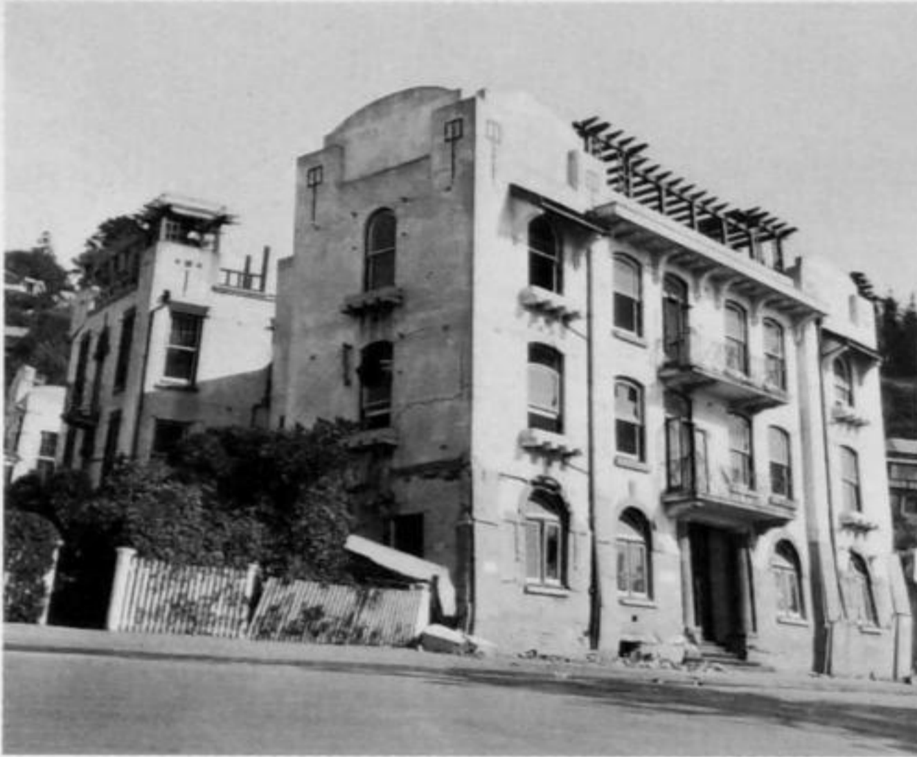
Dr Moore's Hospital tilted badly, crushing its mid-section. The damage was the result of excavations for an underground car-park, undertaken without engineering advice.
