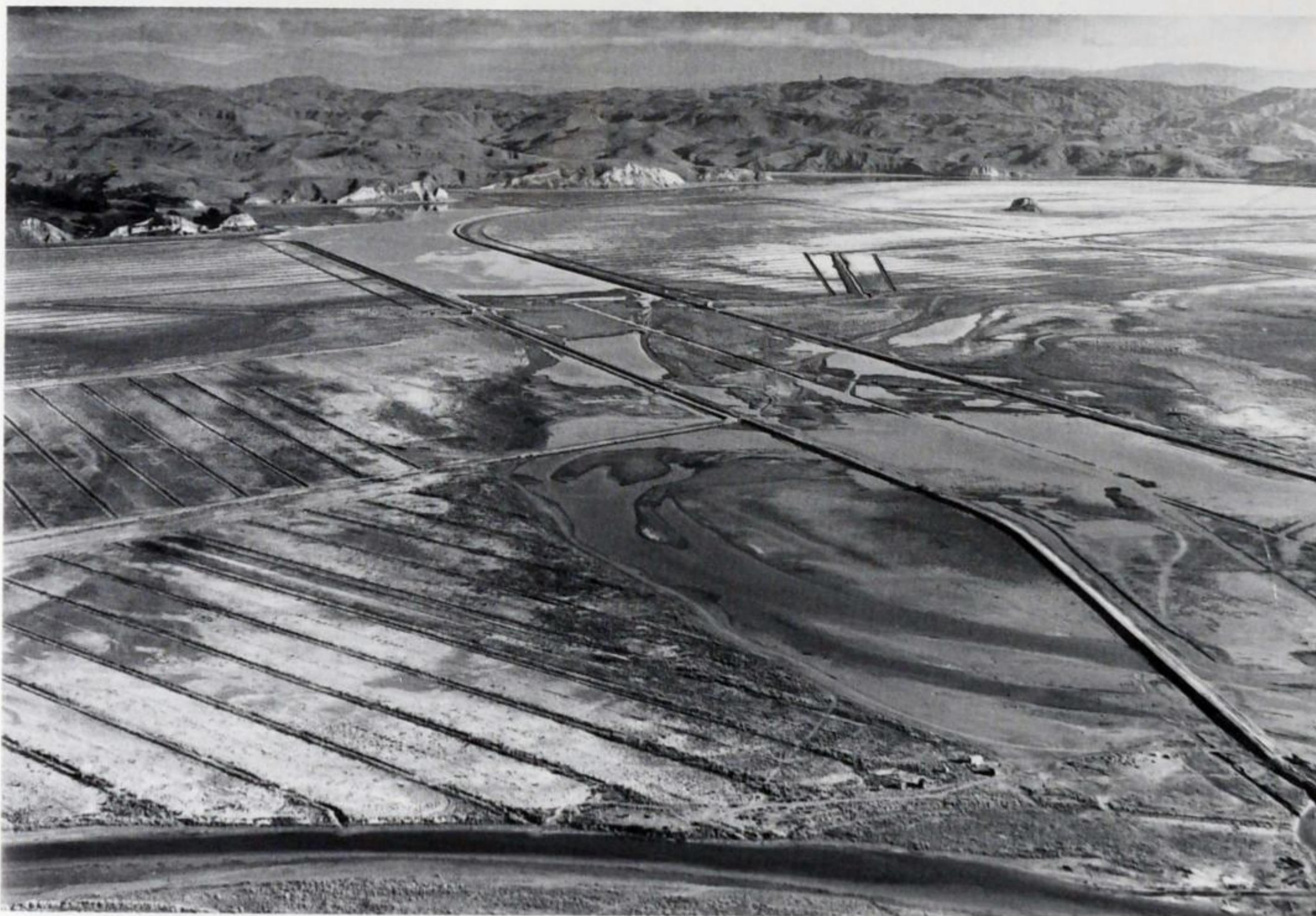
Salt drainage trenches in 1936. The main outfall channel crosses the photograph.
