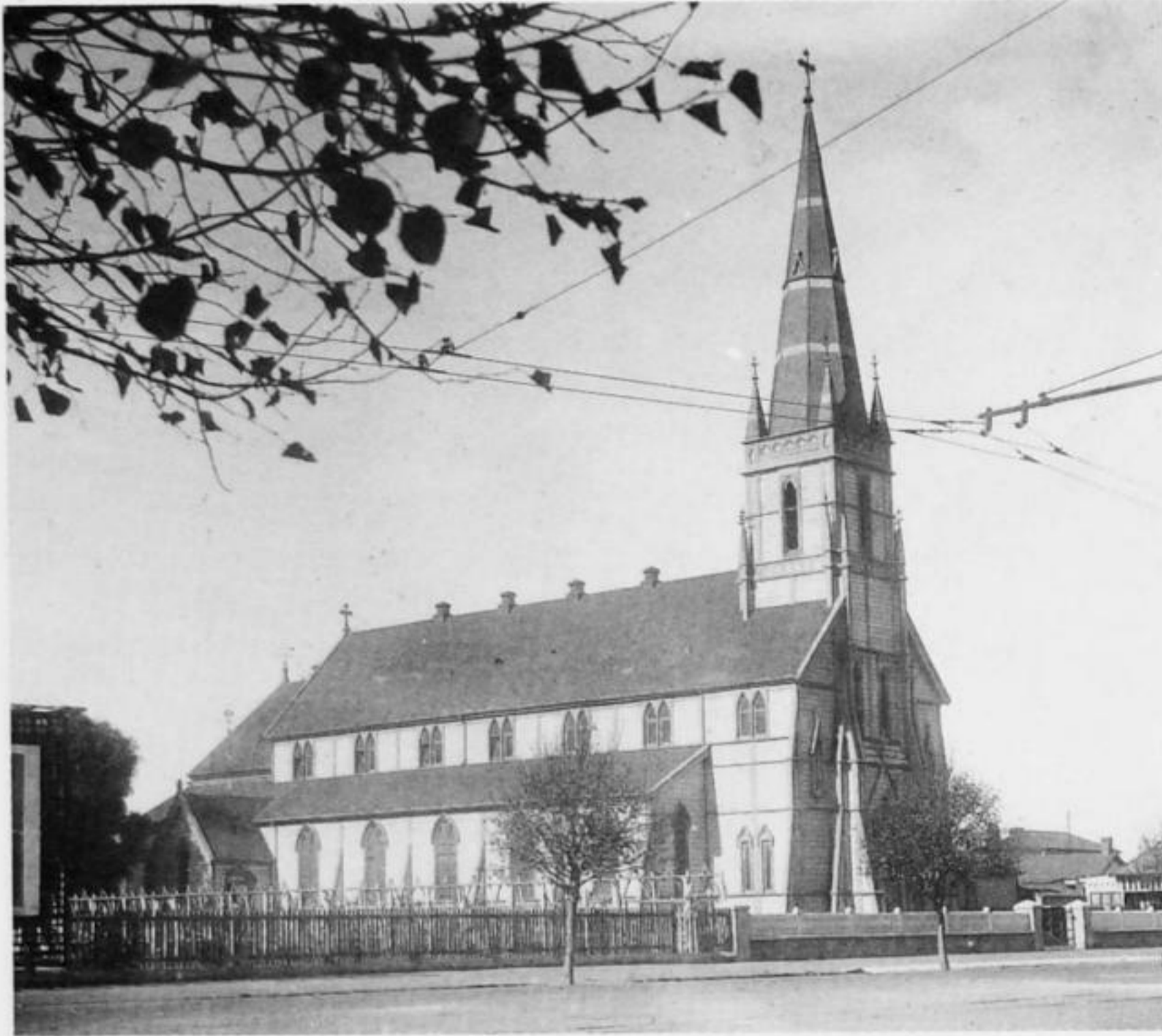
St Patrick's Roman Catholic Church in Munroe Street, built in 1894. It was destroyed by fire one tragic day in 1981.
