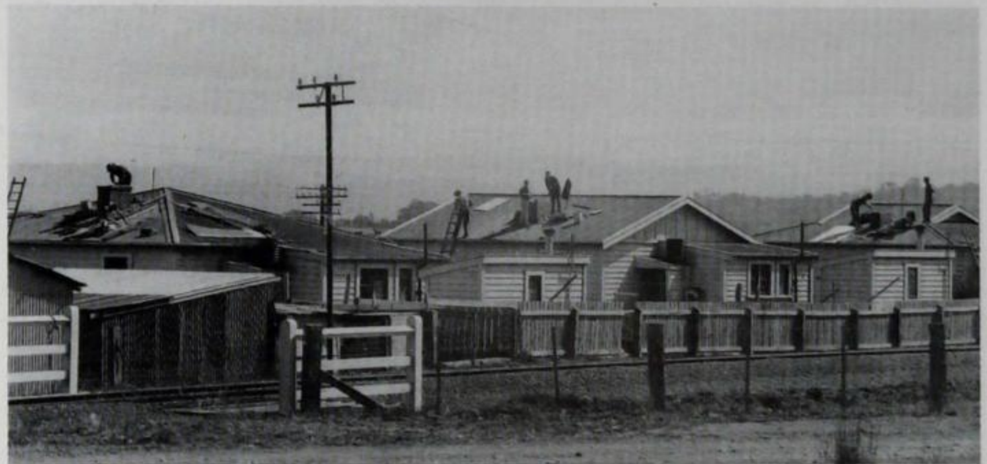
New chimneys being built in Te Awa Avenue, Napier.
