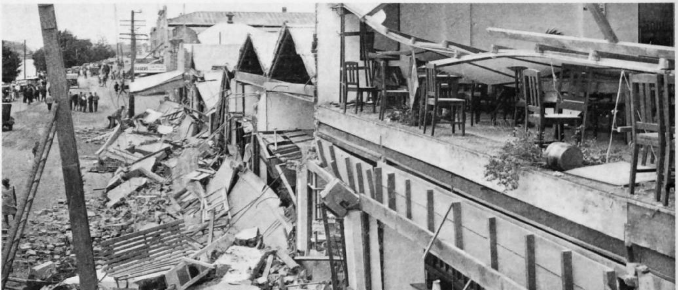
The main street of Wairoa, where considerable damage occurred.
