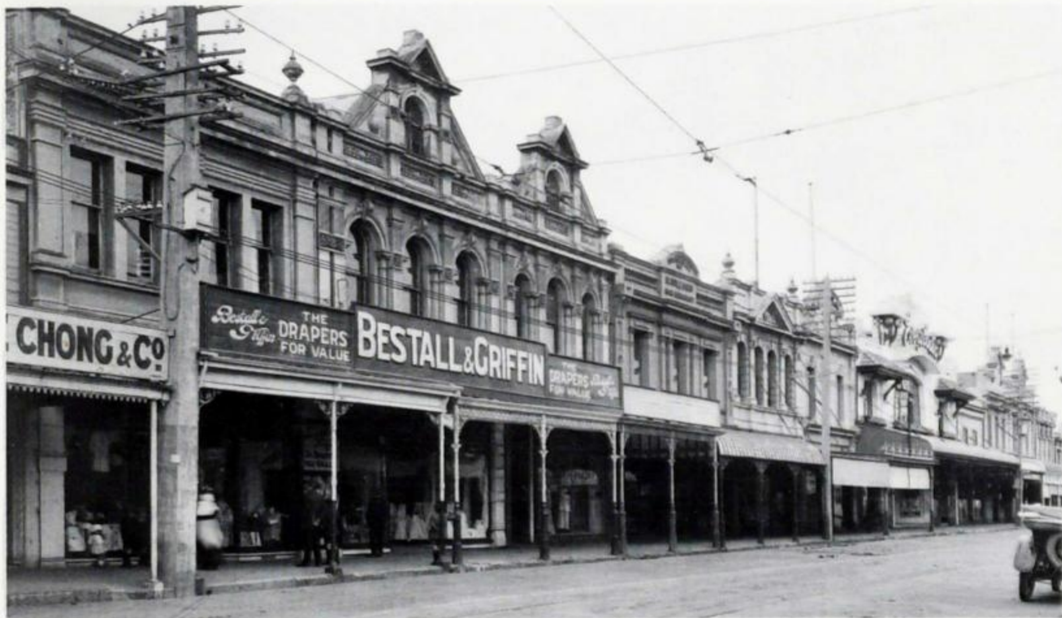
Hastings Street at its curve near Emerson Street. Falling parapets on buildings like these would cause many deaths in the Quake.
