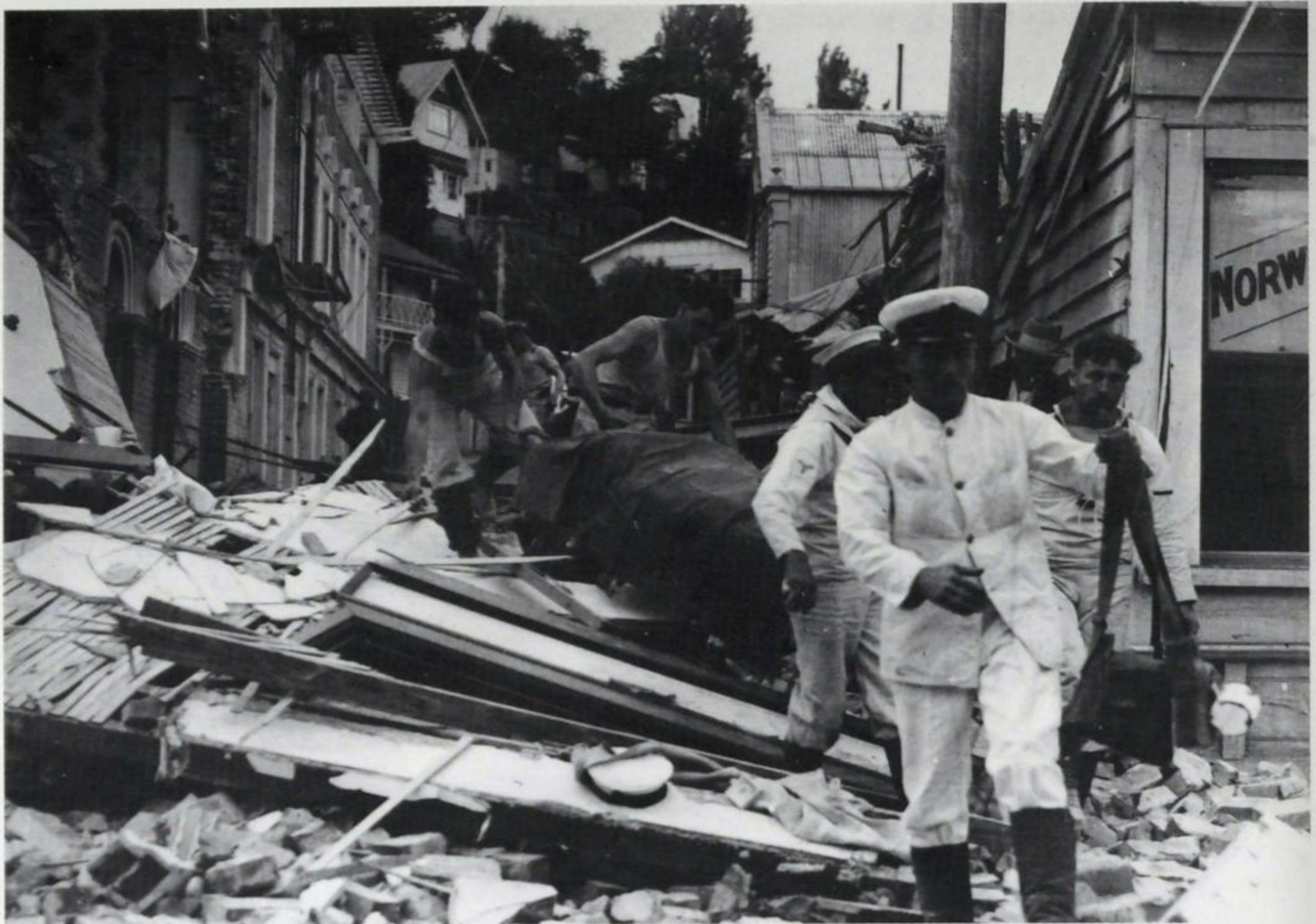
The view up Brewster Street today is very different from this scene, as sailors climb over debris to remove a body.
