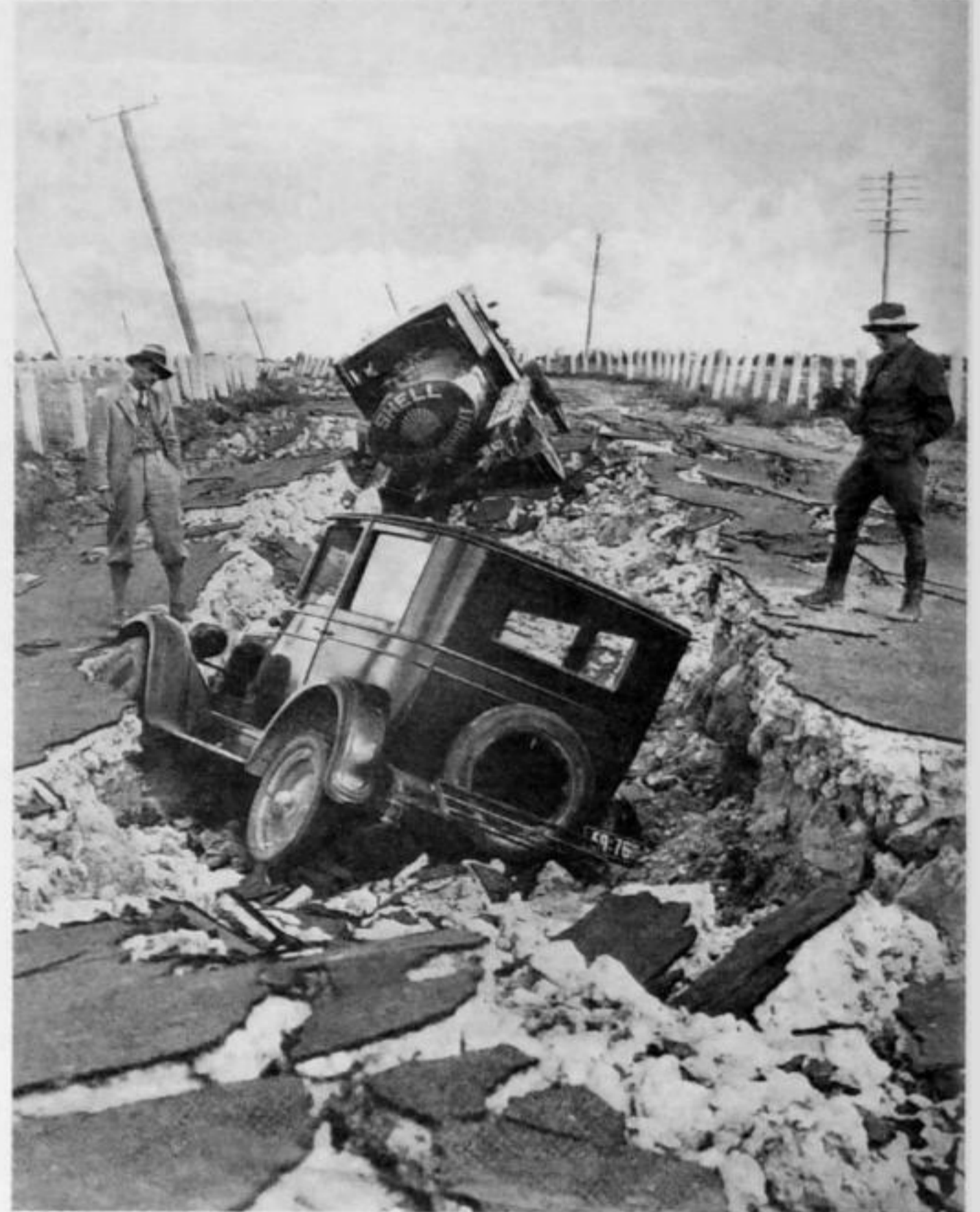
A shock for motorists and truck drivers when the Westshore Embankment Road disintegrated in the Earthquake tremors, because of the unstable silt on which it was built..
