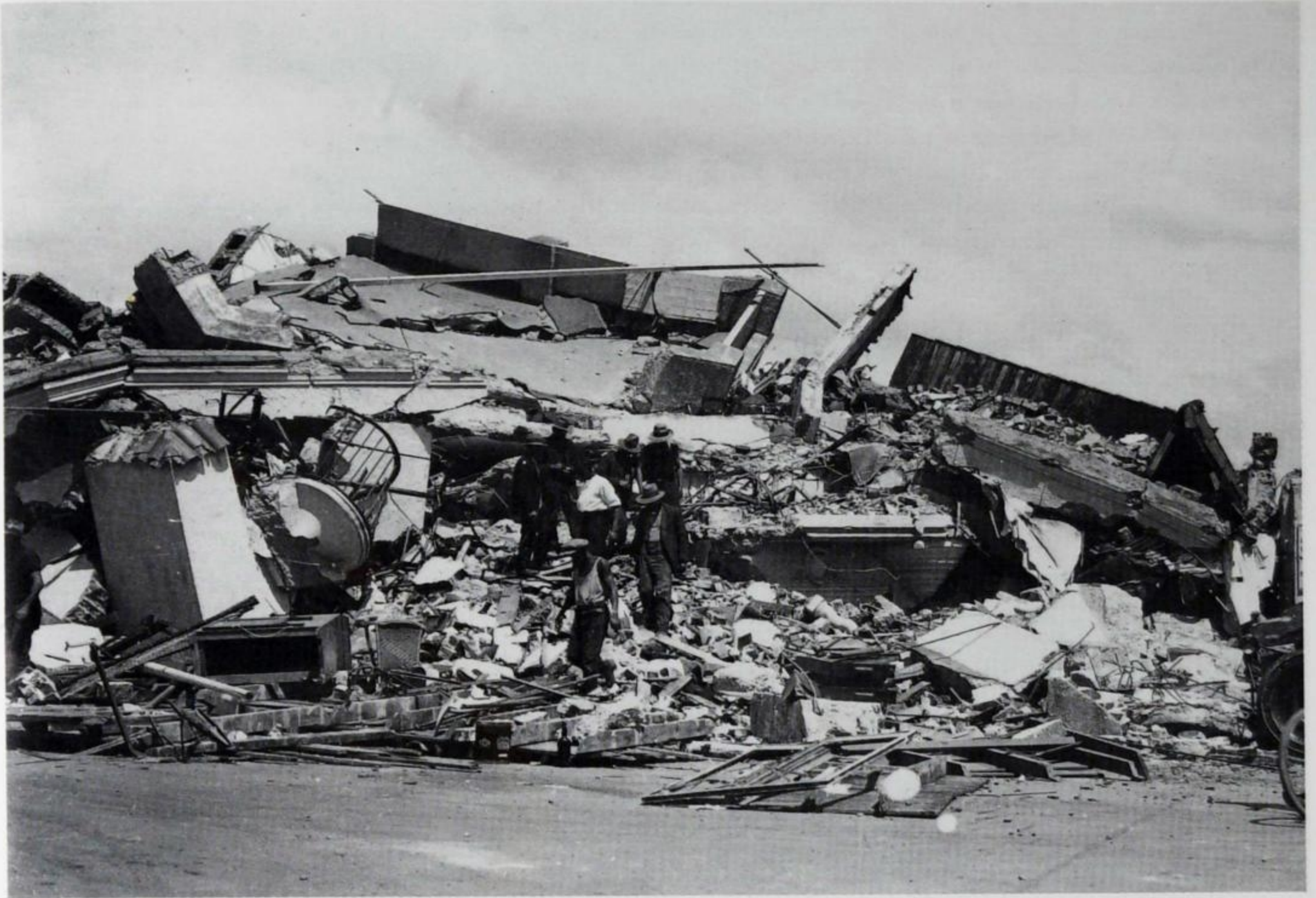
The appalling remains of Nurses' Home, in which several nurses died, asleep after being on night duty. An enquiry into its collapse found it faulty in both design and construction.
