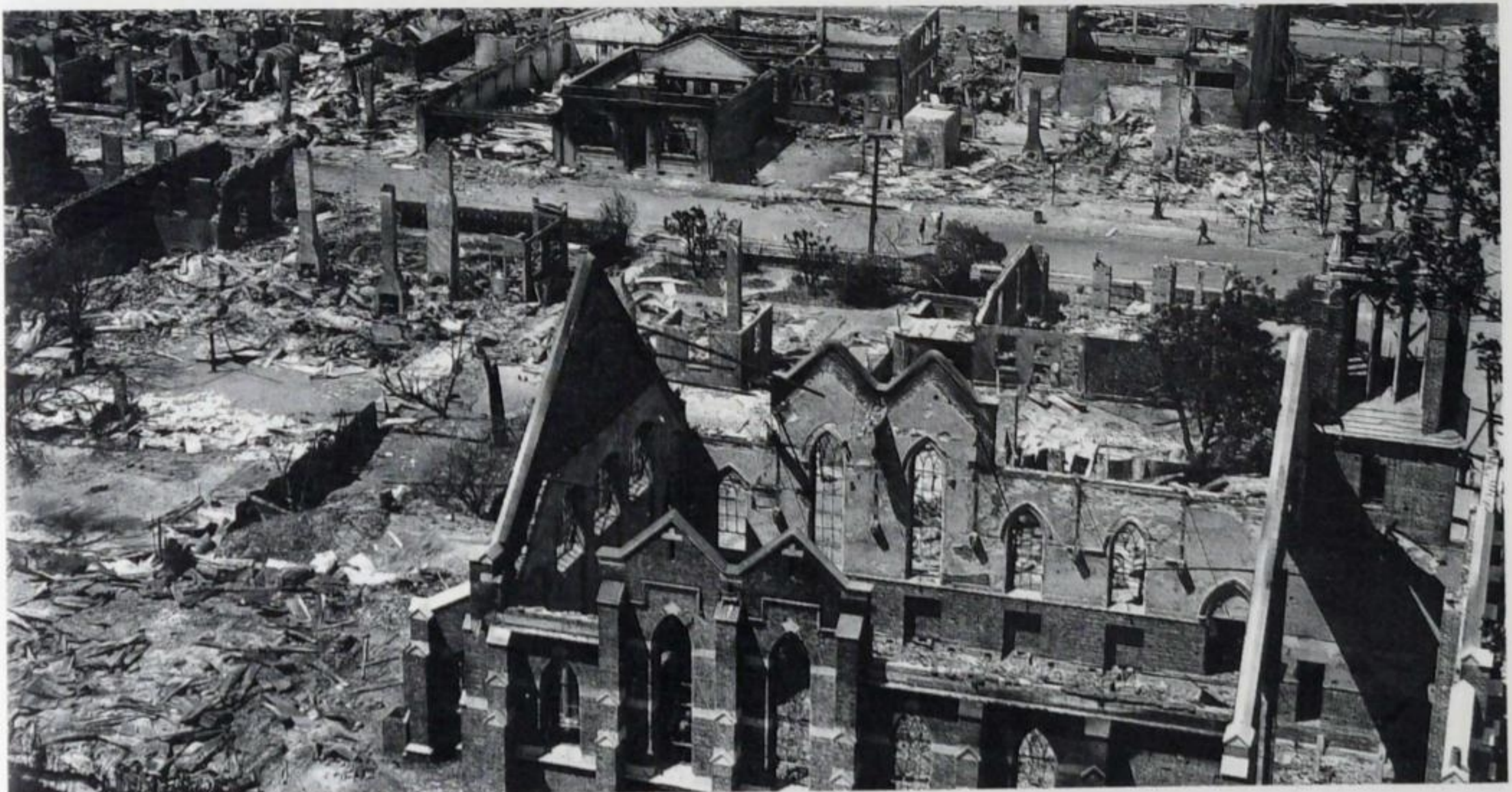
From Tiffen Park, the view over the charred shell of St Paul's Church shows the extent of the devastation in the business area.
