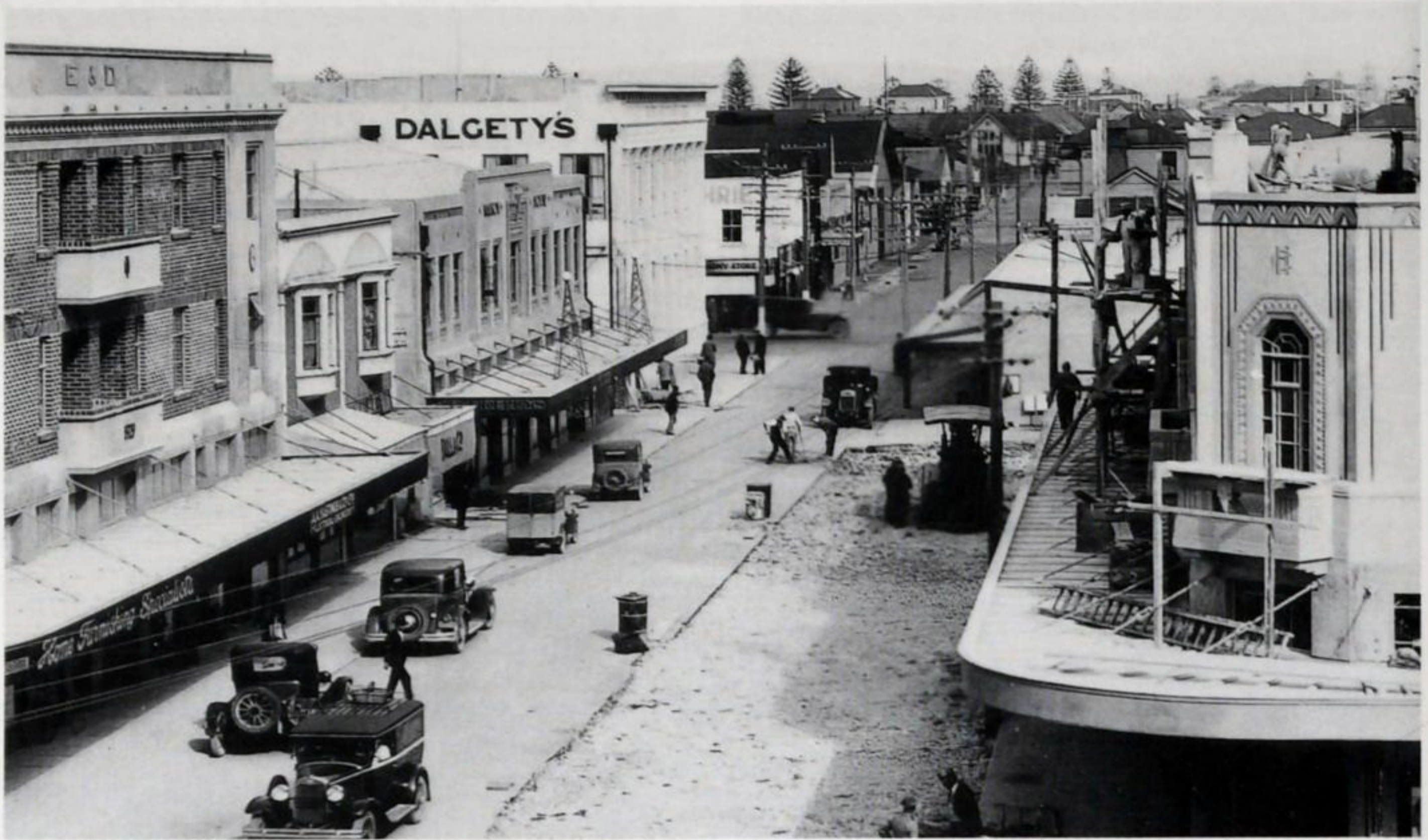
Finishing touches in Dalton Street, with the new Hotel Central at right.
