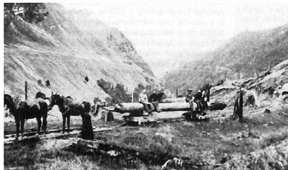
ABOVE: Equipment loaded on to log bogies during the process of shifting Edkin's mill at Whetukura to a new site in 1906. The boiler at the right formed part of a log hauler. (From the A. C. Bellamy Collection)
