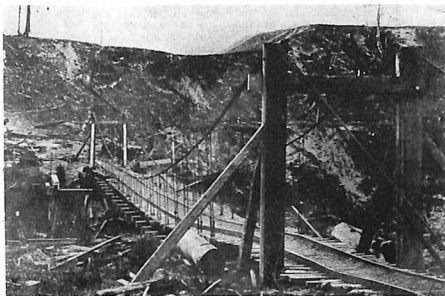
LEFT: The use of swing bridges by railways or tramways is rather rare, but here is photographic evidence of an example on one of Gamman and Company's bush trams in the Dannevirke district. One wonders at its stability under a heavy concentrated load! (From the A. C. Bellamy Collection)
