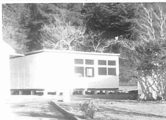
New relocatable classroom.
