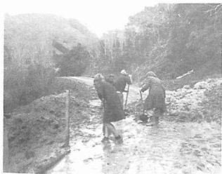
Carol Hopkirk, teacher helps to clear the slip at Tutu Bend.
