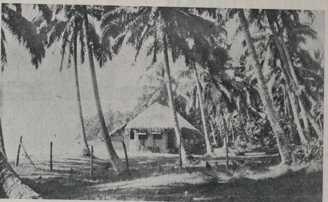
A SOUTH SEAS TRADING OUTPOST.—The home of a French trader in Tahiti. French residents in Polynesia frequently adopt a modified form of the traditional native style of building. The result is a house at once cooler, more airy, and more picturesque than the iron-roofed dwellings to which Britons in the Islands still cling. (Daily Mail Staff Photo)
