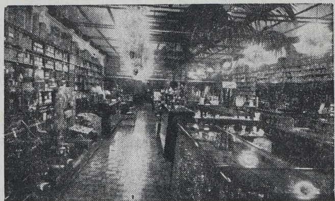
Two views of the premises of Messrs Henry Williams and Sons Ltd., hardware store in Hastings Street. Built in 1933, the shop is one of the most attractive in Napier. This progressive firm was founded in 1862 and with a branch in Hastings does an immense business in both retail and wholesale hardware.
