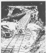
A The bridge was constructed on land then nosed out over the river with a light Bailey Bridge outrigger and a weighted tail. The view from behind. Supported by a line round trees on the H.B. side the new bridge approaches the bank.
